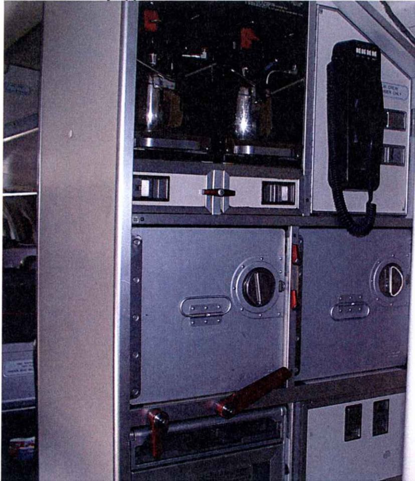
Picture Aft Galley upper section:
